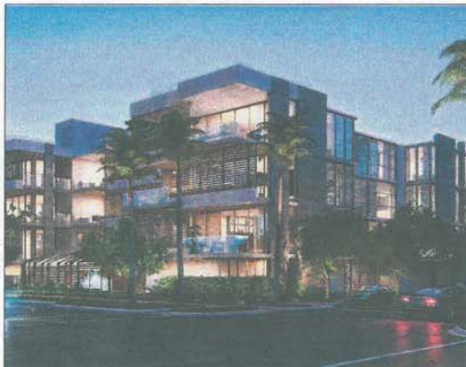
ON SOUTH BEACH: A rendering of Louver House by the Related Group. Its outdoor living rooms are 700-square feet.
